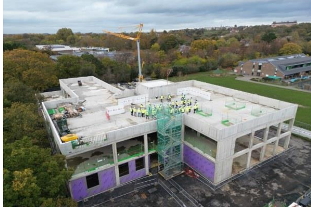
1 - The building is taking shape!
